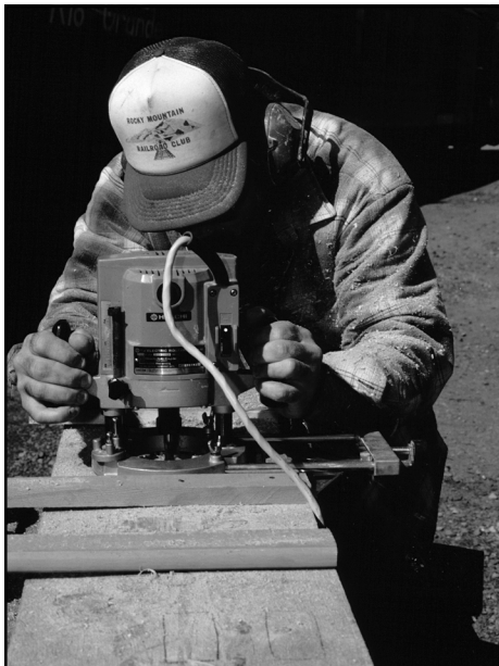
Duane Fields generates lots of dust as he routs out the mortises on the new caboose buffer beam. – Photo © Steve Mason
