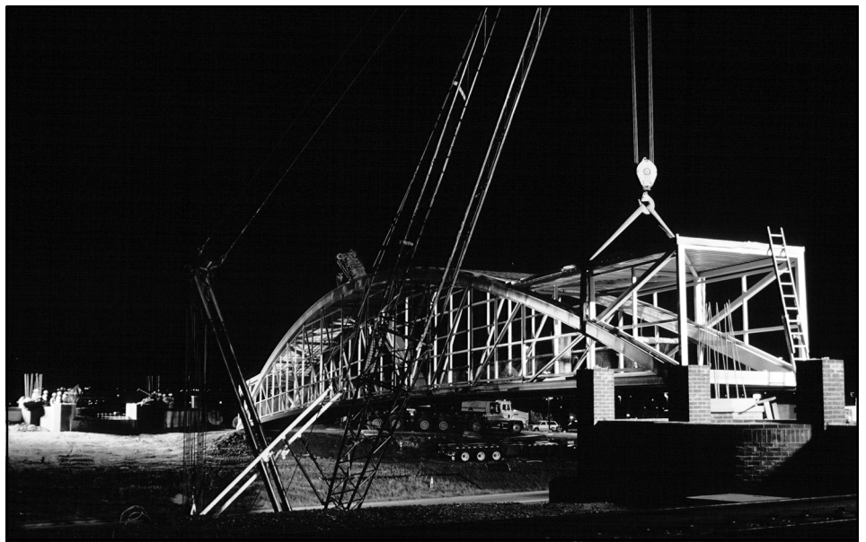
Sure to become a local landmark, RTD's pedestrian bridge over South Santa Fe at Mineral Avenue was placed onto its footings at 1:48 AM on April 17th. All passengers using the Park n' Ride at this southernmost station will use the structure to reach the Light Rail Station. – Photo © Darrell Arndt
