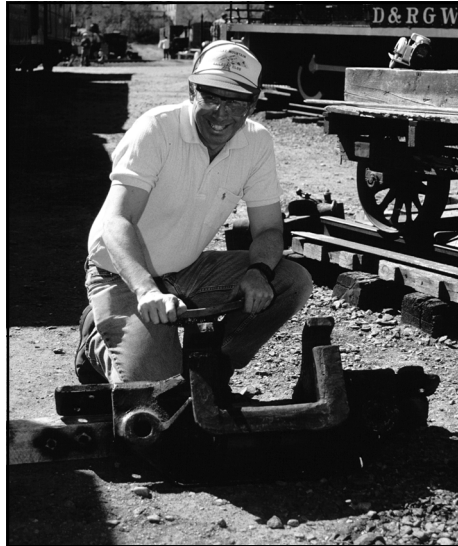
Ken Gow wire brushes the buffer casting prior to painting. – Photo © Steve Mason
